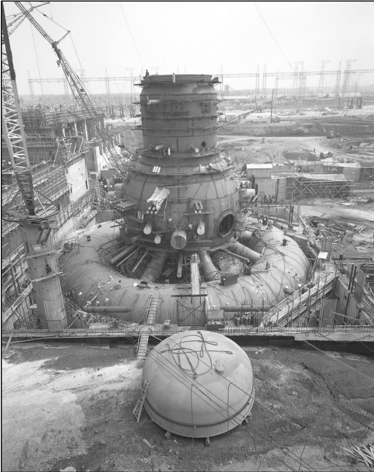
Construction of Browns Ferry Unit 1
